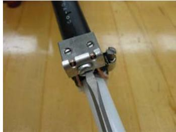
Figure 2 – Insert 10-24 screw through wire retainer and fasten to bonding block.
